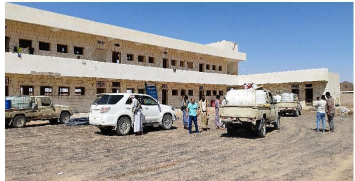
Figure 2: Al Jawfa' school in Al Raiyan sub-district, Khab Wa Ash Sha'af, Al Jawf. Source: HUMAN ACCESS, Nov.2023.
